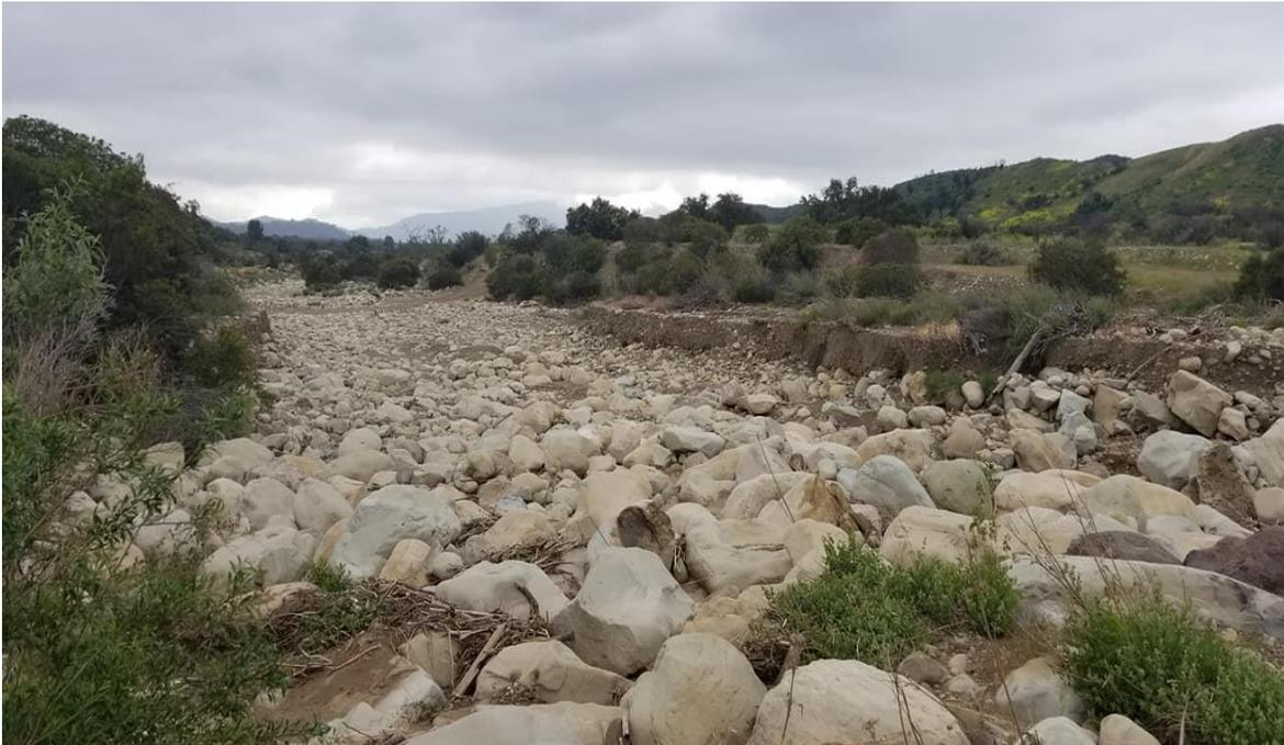
**Photograph 2** View looking downstream of the forebay area and timber cut-off wall. The Ventura River channel banks have sustained heavy erosion from storm events. Sediment removed from the forebay will be used to restore the channel banks (April 16, 2019).
